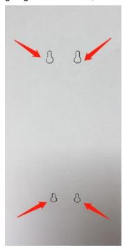
Step4. Follow the marked hole location, drill four holes using 6mm drill tip and nail in four plastic wall-mount nuts into the holes, then mount the G4202TCP on the wall with four wall-mount screws.
